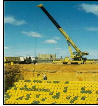
Figure 3-11: Placement of Low Level Waste steel drums at Vaalputs
