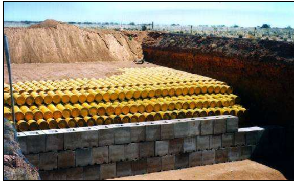
Figure 3-10: Low Level (steel) and Intermediate Level (concrete) radioactive waste drums (respectively above and below) at Vaalputs. The drums are covered with layers of clay.
