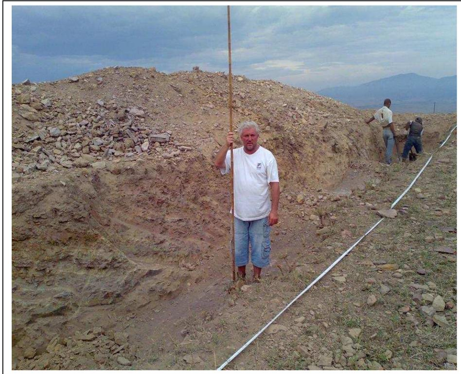
Figure 4 : Trenching conditions in Bokkeveld shales. Onset of heavy ripping conditions for rock excavation at approximately 1.5m.
