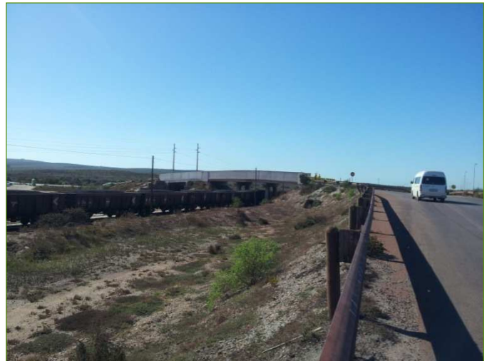
Figure 5: Photograph of the Duferco Bridge
