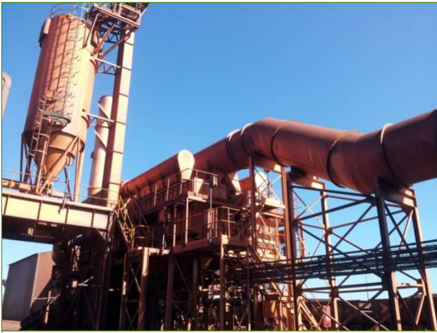
Figure 4: Dust extractor on existing tippler
