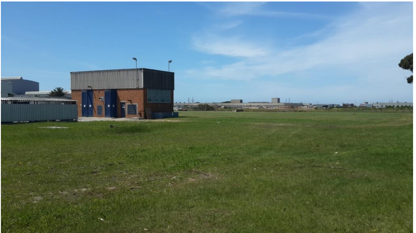
Facing south east
