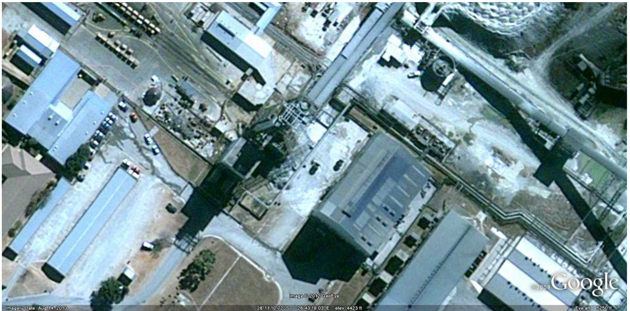
Figure 2: Aerial photograph of the Gold Fields Beatrix Mine Indicating the Proposed Location of the Co-generation Plant (not to scale)
