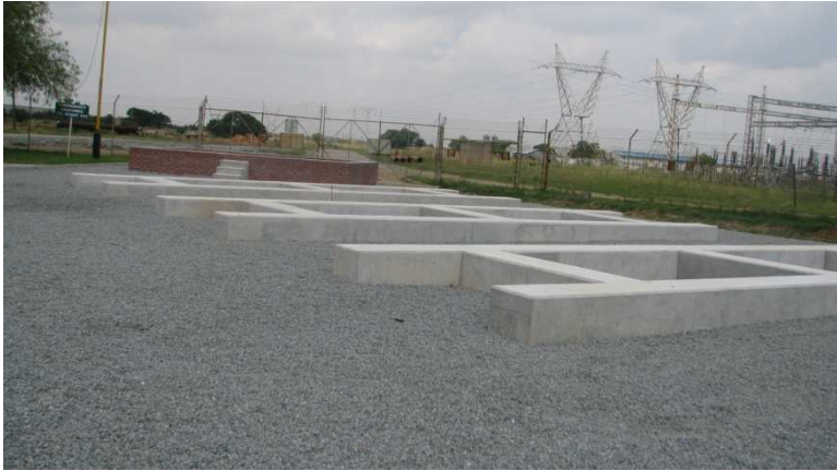
Figure 9: Shaft 1: Existing Facility at Beatrix
